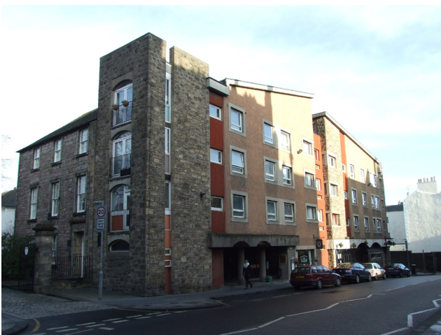
© EWH. Energy Efficiency for Post-War Listed Buildings.
